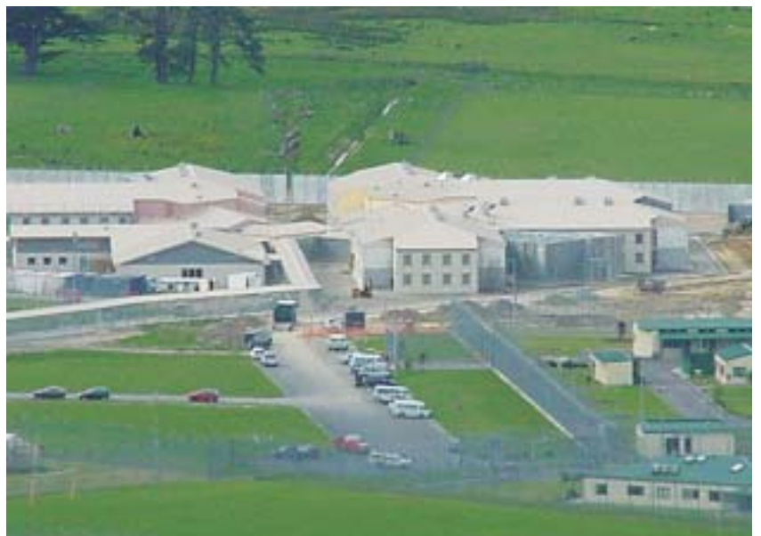
Part of the $43m worth of new facilities.
