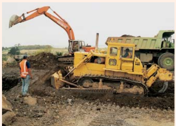
Earthworks are underway to make the proposed site suitable for building
