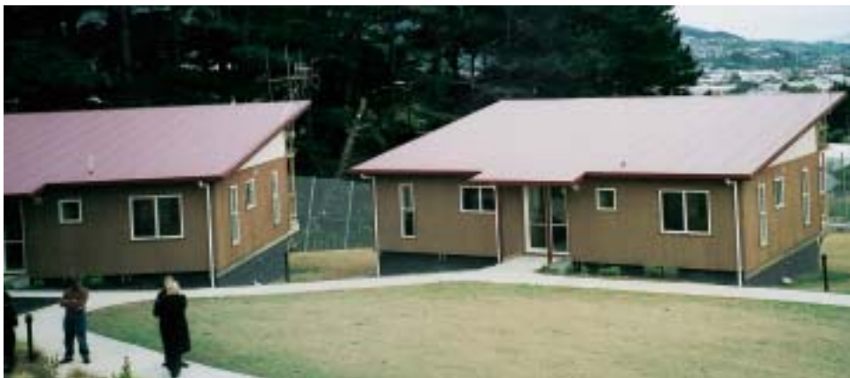
Newly built and landscaped, Arohata Prison's self-care units await their first residents.
