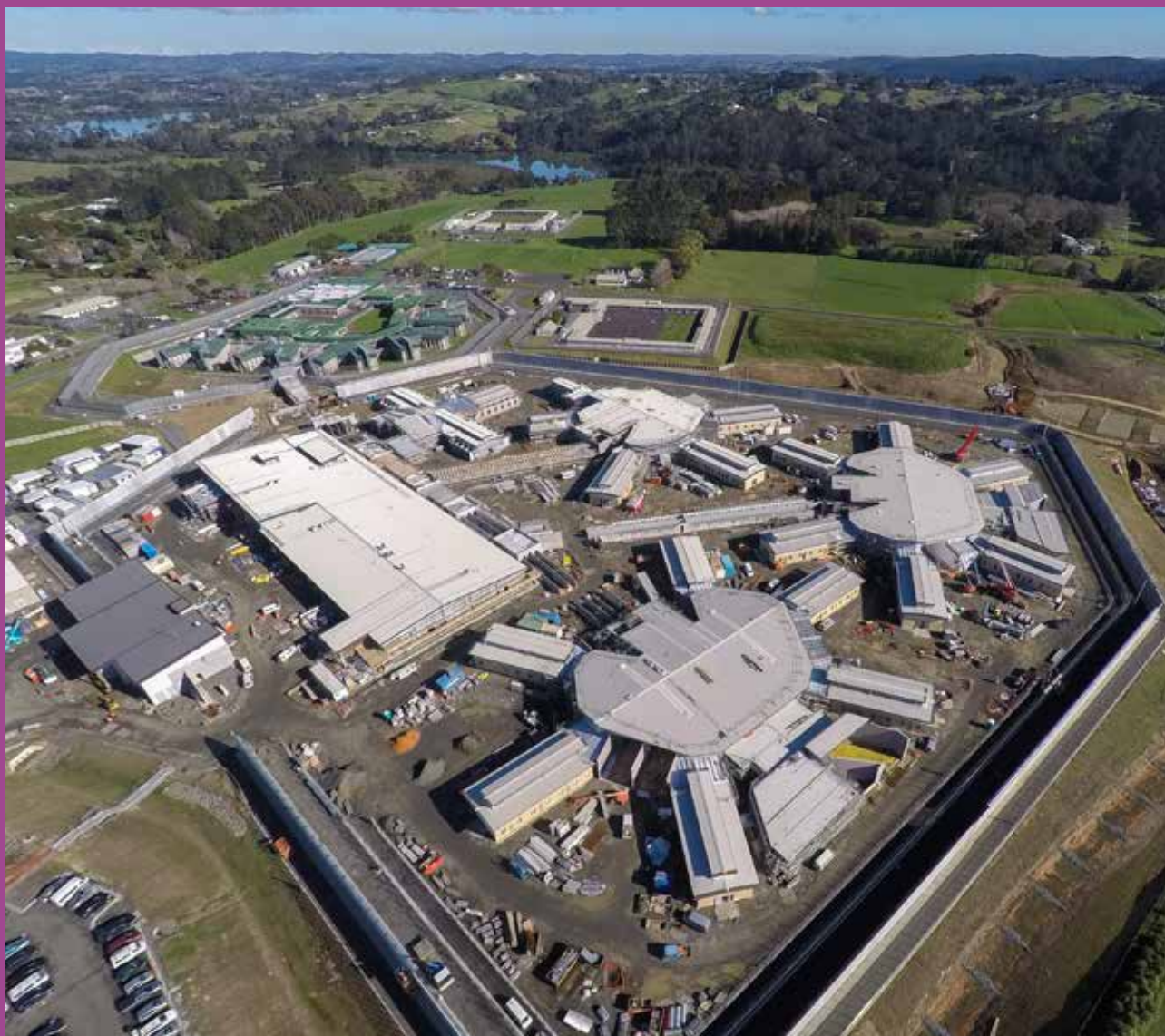
Birds eye view of Auckland Prison under construction in June 2017.
