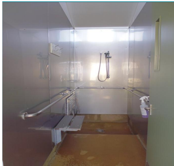
Figure 19: Adapted shower facility - s.6(c)
